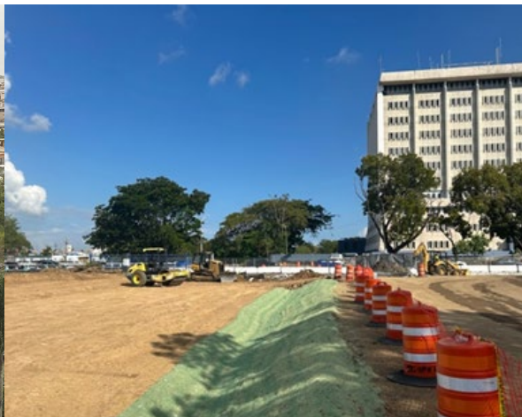
Rio Puerto Nuevo CNT-2 Roosevelt Bridge Replacement
